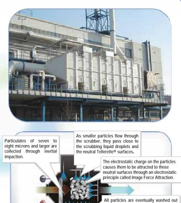
All particles are eventually washed out of the scrubber with the exit liquor. Noxious and malodorous gases are absorbed and reacted in the same scrubbing liquor.
